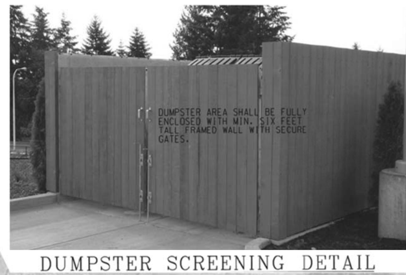
DUMPSTER SCREENING DETAIL
